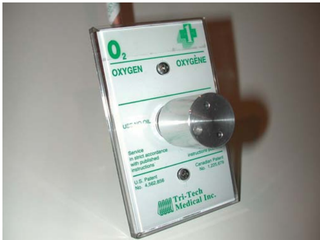
DISS Gas Outlet with DLO Locking Device Installed
